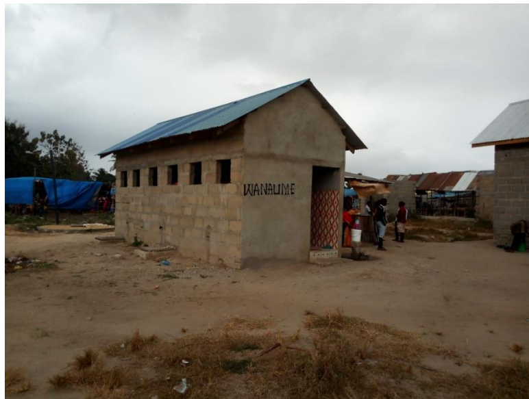
Figure 4: Public toilet at the project site
